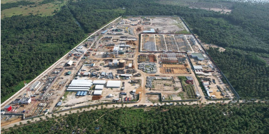
Atinkou thermal power station under construction
